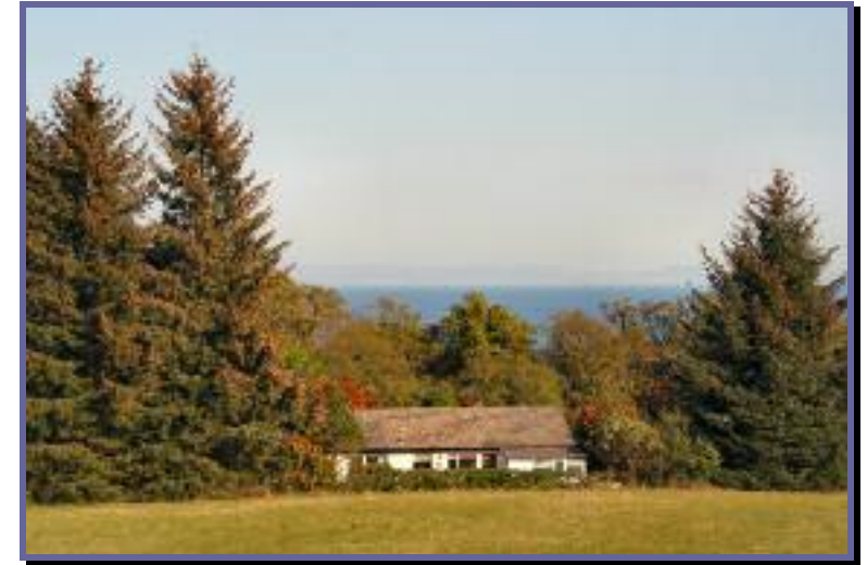
View of Kelvinedge from the rear
